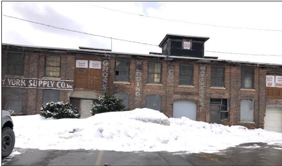
Photo 6: Rear side, photo taken on 2-20-20
